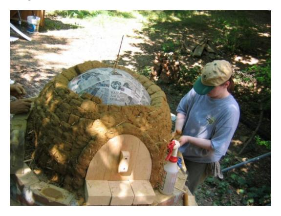
We have featured tutorials on DIY clay ovens and pizza ovens before (use the K.W.N search facility and search - oven). The difference with this tutorial is that the oven is made largely for free, using natural materials such as clay, straw and earth. The only real cost is for the bricks for the base, but even these could be scavenged for free, there are always old bricks to be had for free if you know where to look.
