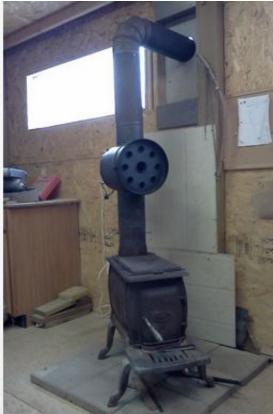
If you have a small woodstove in your home or workshop etc, fitting a heat exchanger on the chimney is a great way to reclaim the huge amount of heat which is lost up the chimney. You can purchase ready made heat exchangers, but they usually cost in the region of \$200. If you are a proficient DIY-er and you are up for a bit of welding, you can build your own heat exchanger for a fraction of the price.
